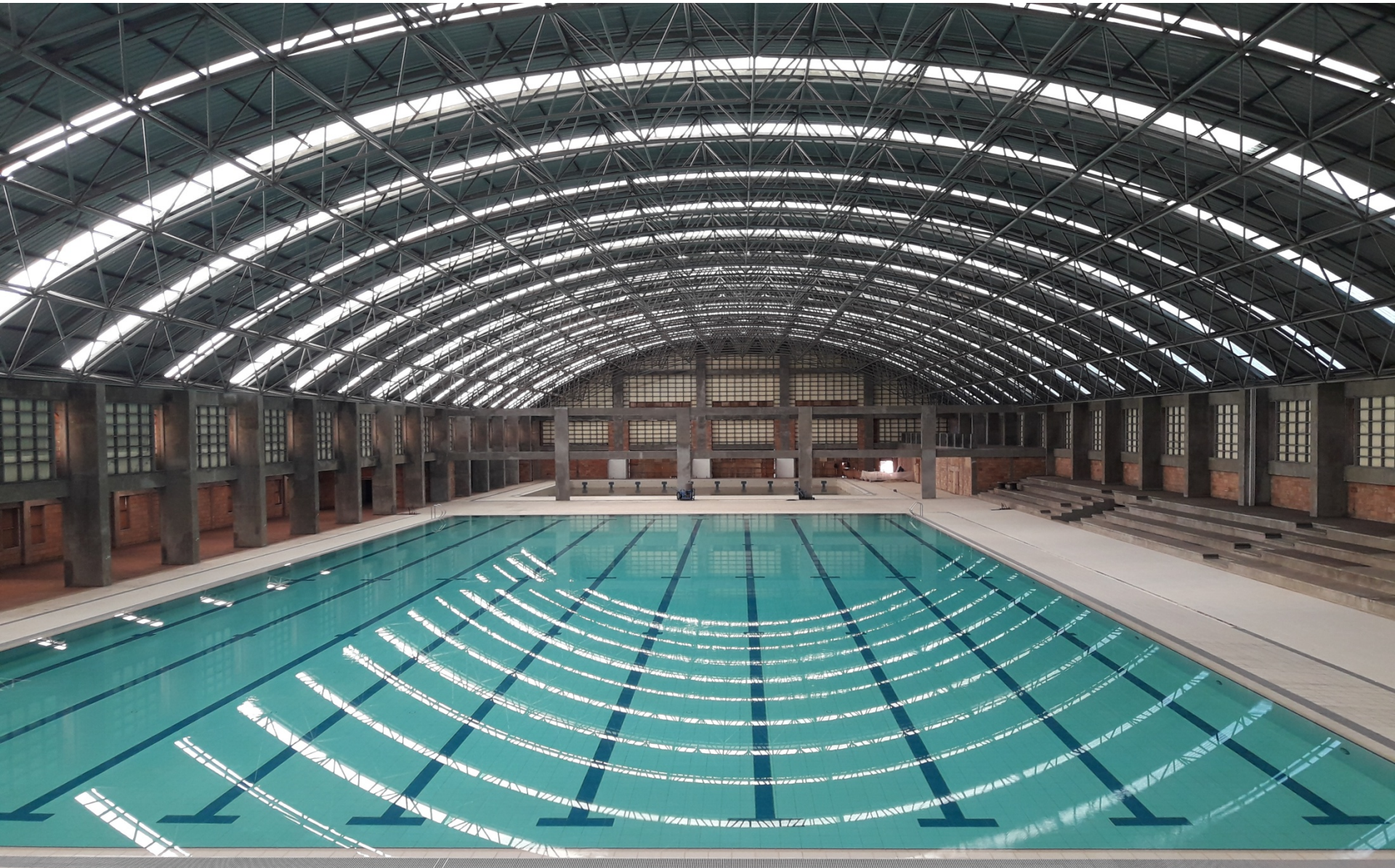
Olympic-size covered swimming pool
