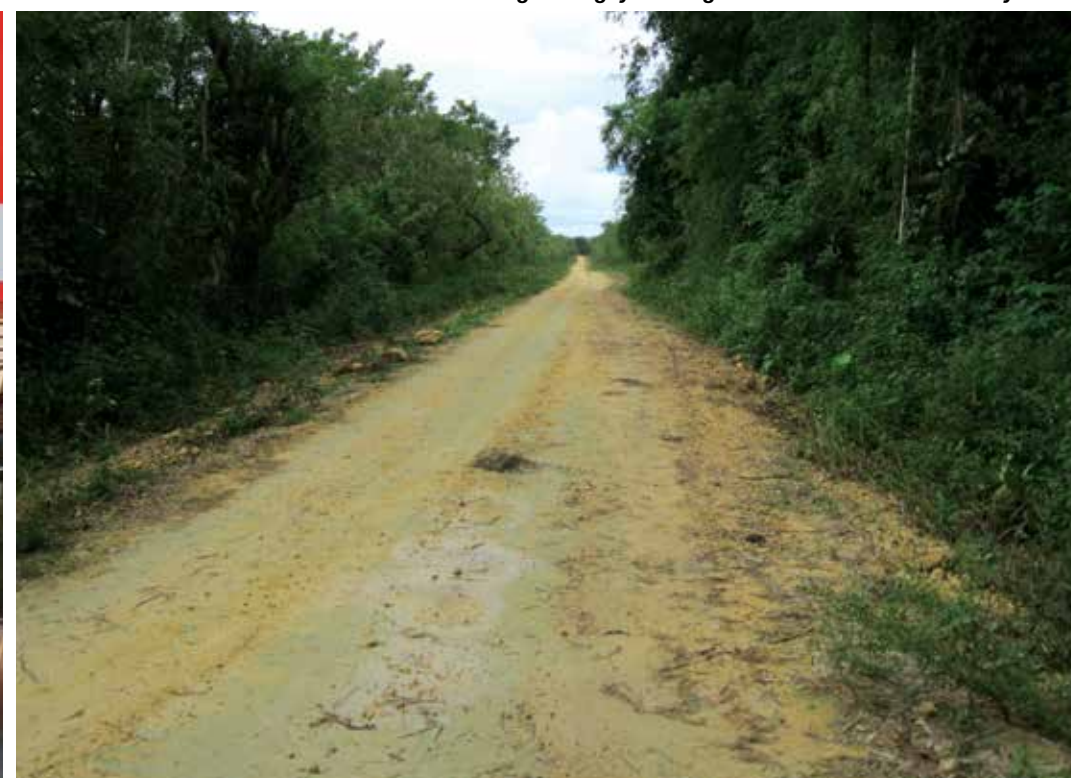
Connecting barangays through road rehabilitation on Sibay Island
